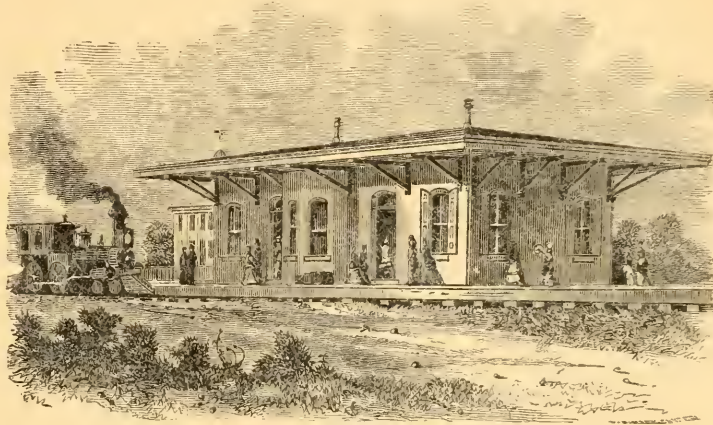
STATION, CENTRAL RAILWAY OF NEW JERSEY.
